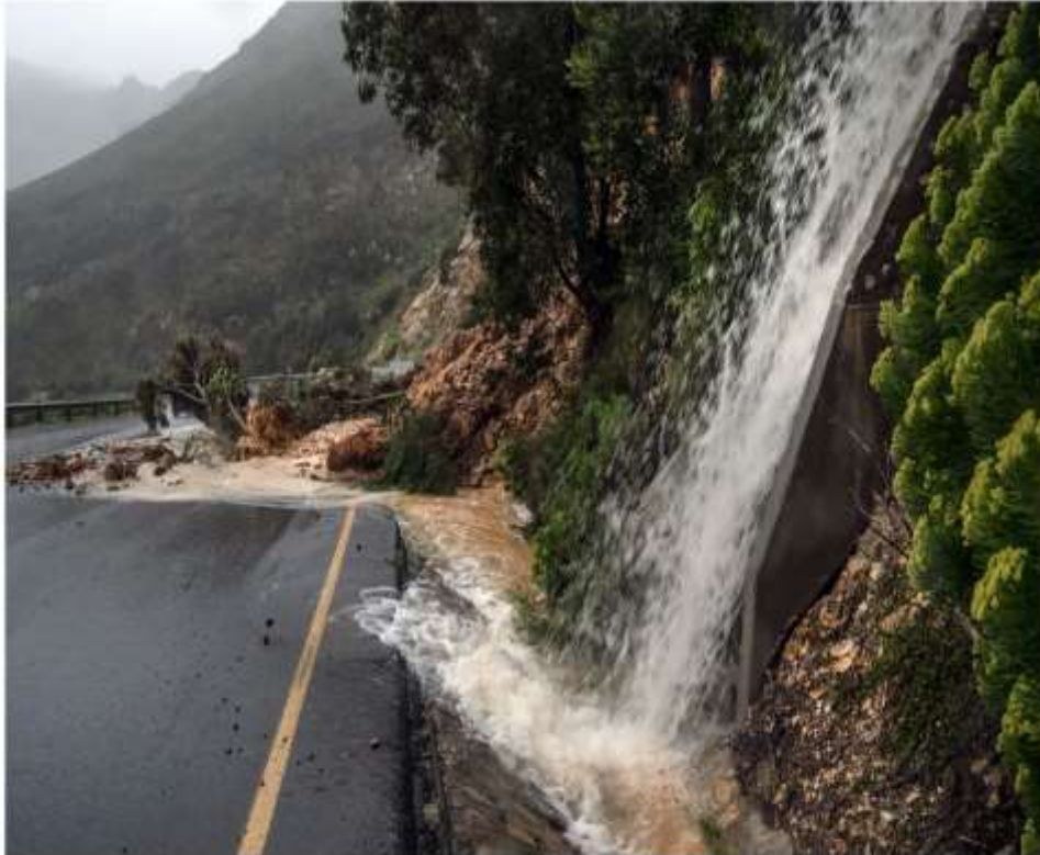
Sir Lowry's Pass above Somerset West was closed for hours due to fallen trees on 25 September 2023. Disaster management officials have been working round the clock amid reports of flooded roads, damaged homes, uprooted trees and power outages. (Photo: Benton Geach / Gallo Images)
